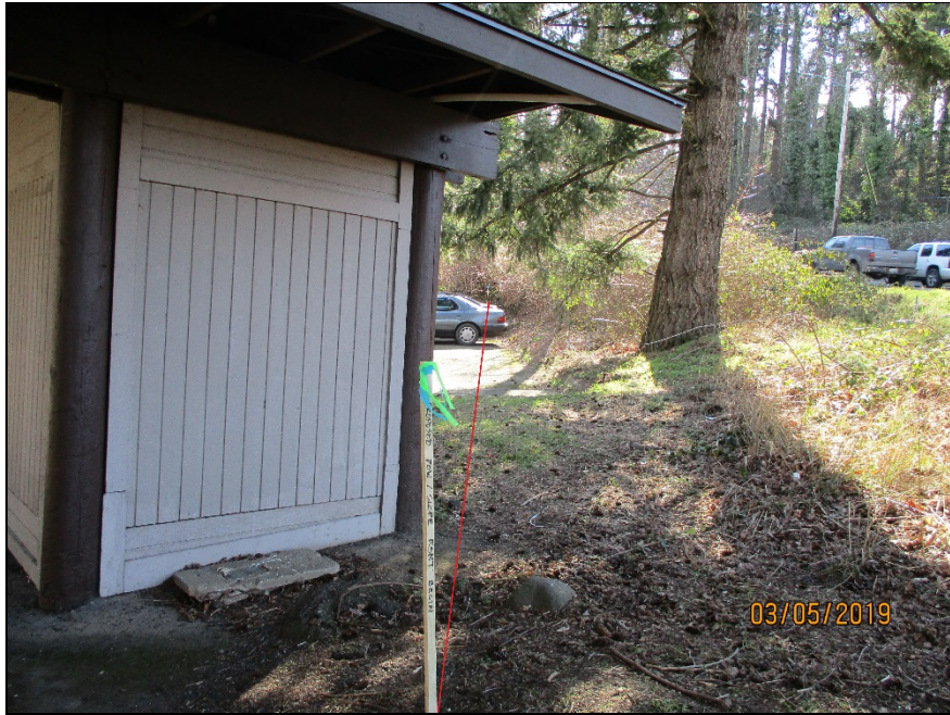
Corner of carport that is in permanent easement area.
