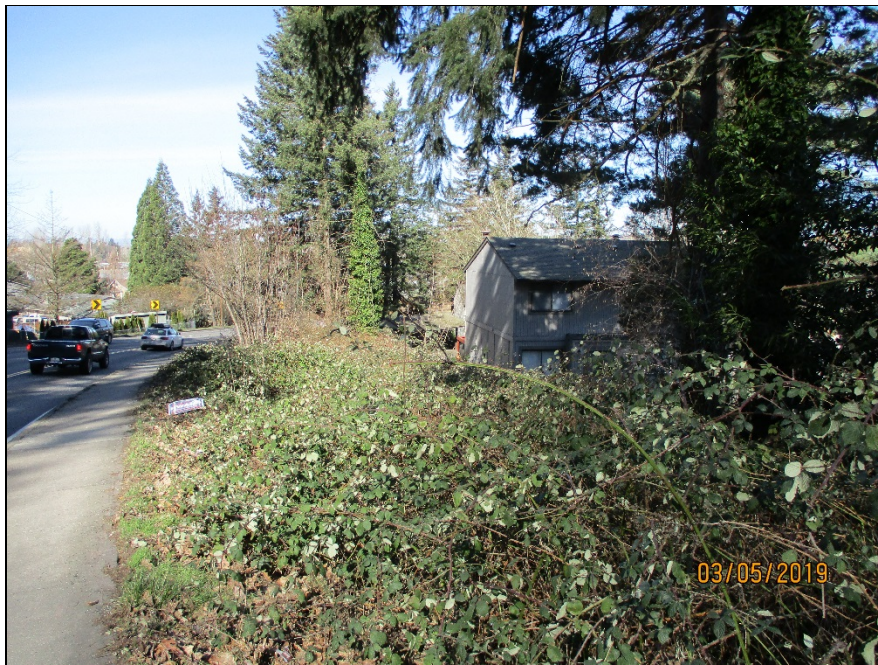
View looking northwest. Building next to where retaining wall will be installed.
